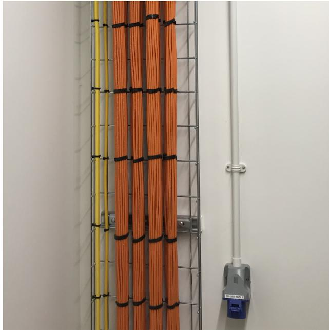
**Figure 4: Cable Contained in Cable Basket**
