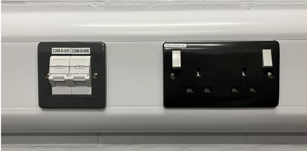
**Figure 5: Double Network Socket with Power in Dado Trunking**
