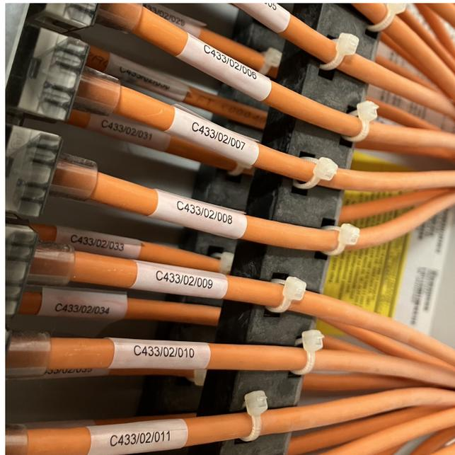
**Figure 17: Cables Labelled at Patch Panel**
