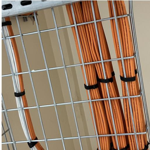
**Figure 6: Horizontal Network Cable Basket**
