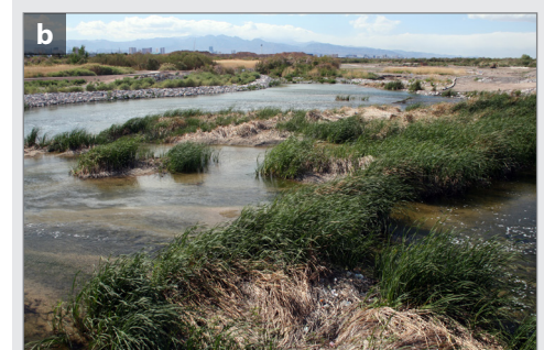
Figure 23. Example illustrating the use of constructed wetlands to manage flash floods: a) the Las Vegas Wash (view looking upstream) showing the deep (4-5 m) erosion resulting from flash floods in the 1980s and 1990s; b) subsequent design and construction of The Wetlands Park Nature Preserve adjacent to the Wash was partly in response to the impacts of this particular geohazard and consists of a series of constructed wetlands that are being actively managed using surface runoff, reclaimed water, and water level control structures. The streams, ponds and plants help restrict erosion and provide habitat for wildlife, while trails and overlooks provide nature viewing and other recreational opportunities. High rise buildings along The Strip in Las Vegas are visible in the far distance (Photographs: Stephen Tooth).
